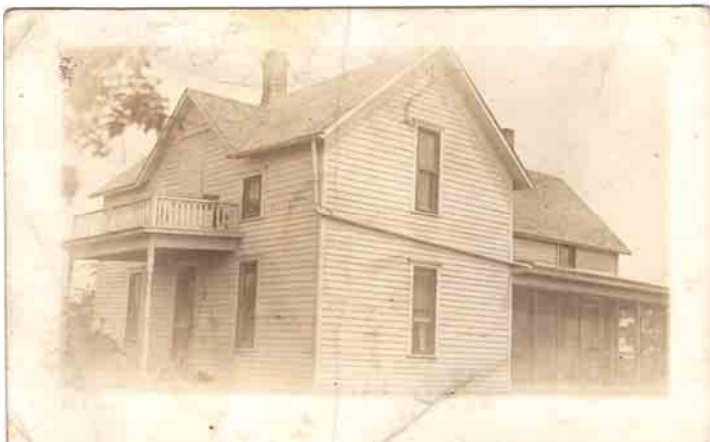
The home occupied by the Henry and Dora Mueggengborg family 7.5 miles east and one mile north of Okarche. The house remained standing until the early 1950's when its later occupant, son Paul, replaced it with a newer structure. It was in this house that the family raised their nine children to adulthood.
